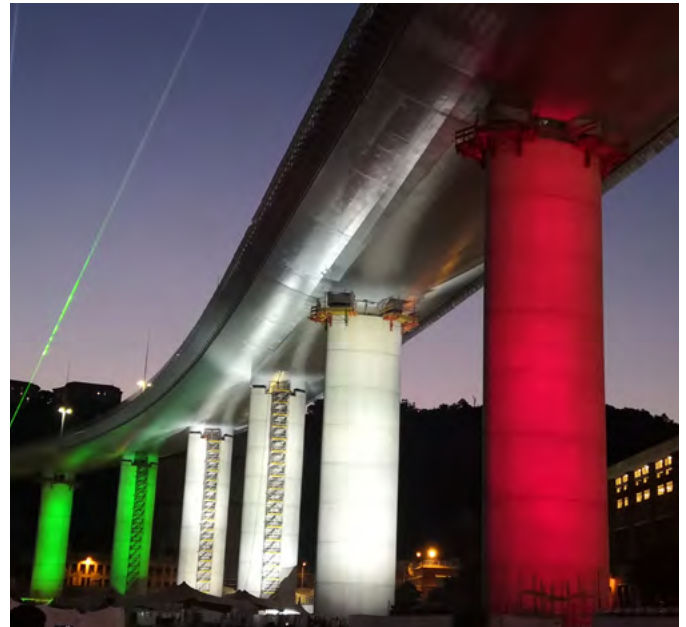
San Giorgio Bridge, Genoa
